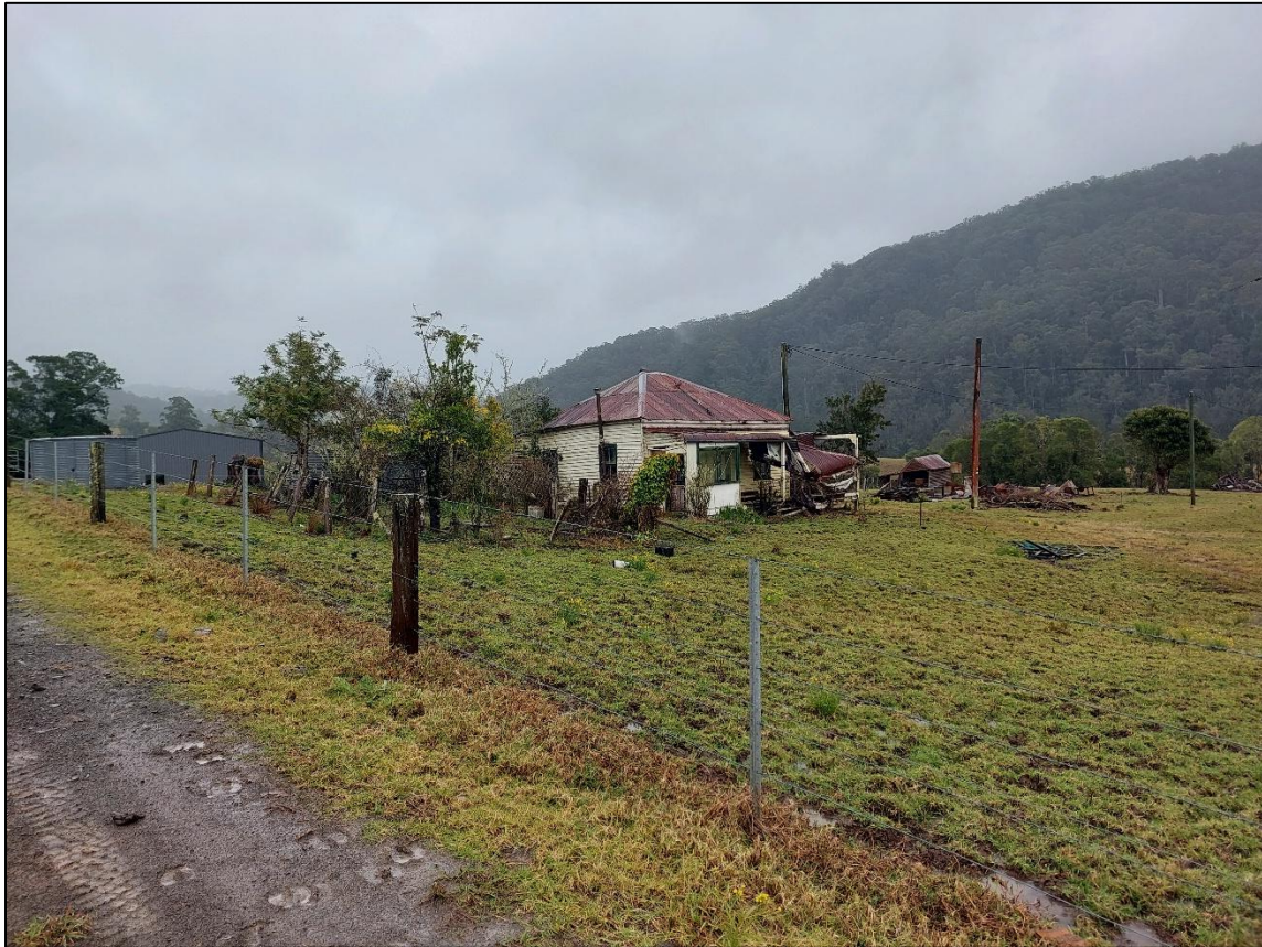
Figure 4 Subject Site looking North west
